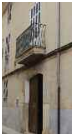
Can Bereiol, the headquarters of the electricity plant (building located next to the electricity tower)
